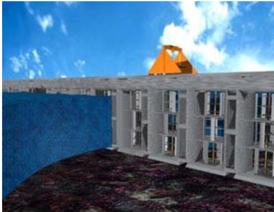
Figure 10-4 Blue Energy's Tidal Bridge With Davis Turbine (Source: Blue Energy)
