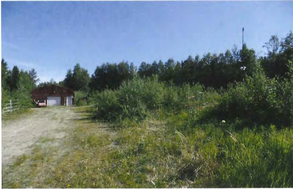
1392 GILMORE TRAIL - LOOKING NORTH ON THE SITE TOWARD THE PROPOSED CELL TOWER LOCATION.
