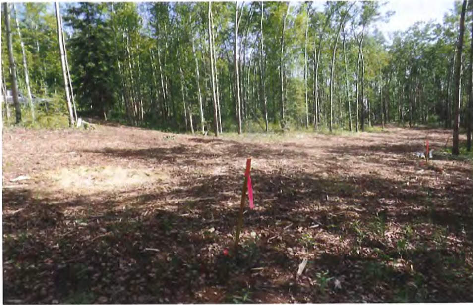
1616 WOLVERINE LANE - LOOKING SOUTHERLY ACROSS THE SITE - THE PROPOSED CELL PHONE TOWER WILL BE PLACED IN THIS VICINITY.
