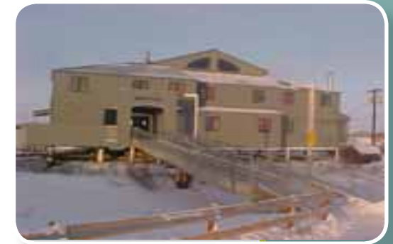
KU 105 John Sackett Residence Hall
