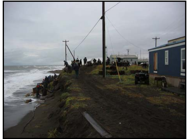
Photo 2: Work crew at eroded shoreline in Kivalina. (Credit: Colleen Swan)
