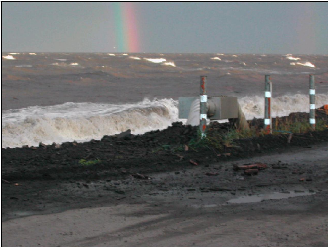
Photo 13: Remains of infrastructure at eroded shoreline in Unalakleet. (Credit Steve Ivanoff)
