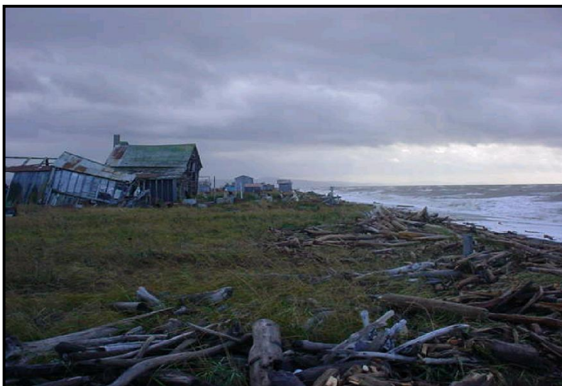
Photo 7: Lot inundation at Shaktoolik. (Credit: Steve Ivanoff)
