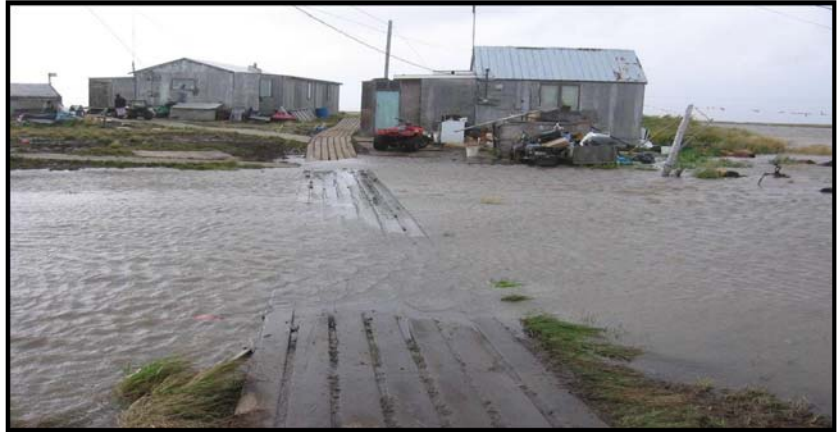
Photo 5: Flooding during coastal storm in Newtok. (Credit: Stanley Tom)
