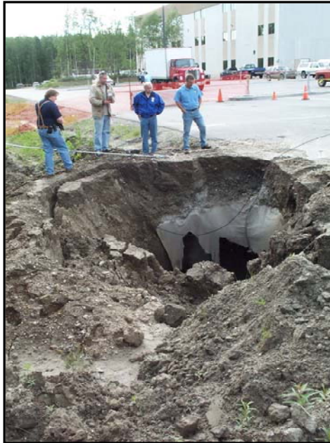
Thermokarst depression on the edge of the Geophysical Institute UAF parking lot (Fairbanks, Alaska). Surface disturbance related to the parking lot construction triggered the permafrost degradation and ground ice melting. This created a subsurface void within the ground. The roof of this void collapsed when surface and ground waters saturated the soils during spring and beginning of summer. Photo by Prof. Vladimir Romanovsky, University of Alaska Fairbanks.
