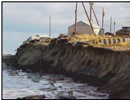
Bluff erosion & permafrost thaw, Shishmaref (c 2002) Kawerak
